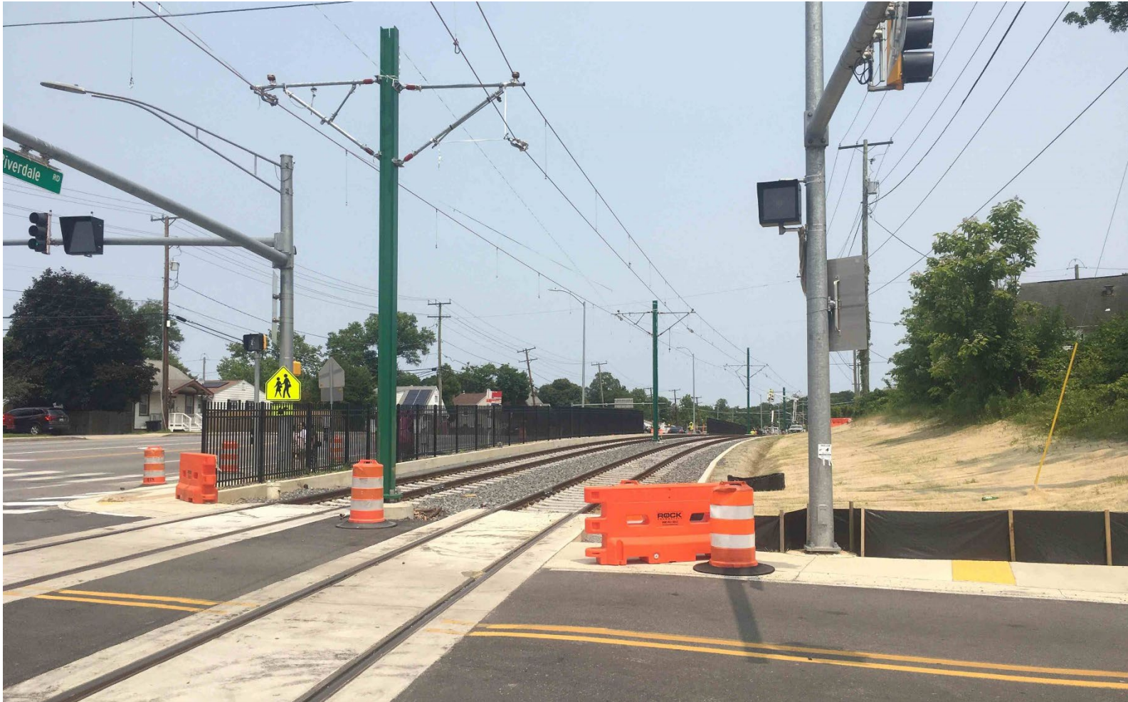
Semi-exclusive side running alignment
